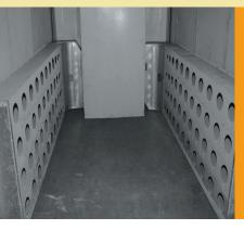
The panels will be insulated with mineral wool bats, 4" thick, when compressed into the panel, will be firmly held to prevent the usual settling due to vibration, Thus avoiding an un-insulated space at the top of the panels through special construction.
